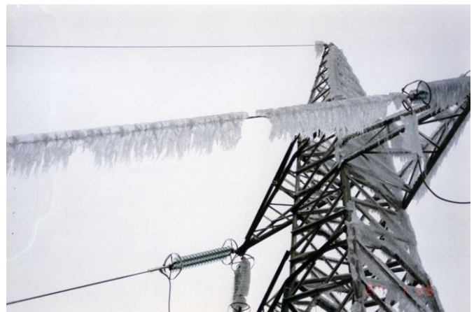
Figure 1. Picture of real Ice loading condition on TERN A 400kV La Spezia-Vignole overhead line
